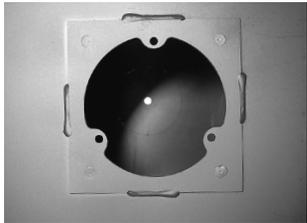
There is now an unblocked view of the smoke discharge. Remove dirt and dust, and mount the parts in reverse order.
